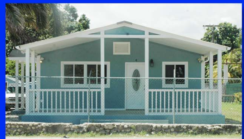
Secure Safe Buildings
