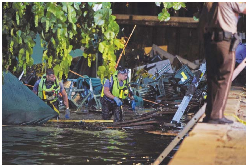
Rescue divers search for missing people after deck collapsed at Shuckers restaurant in North Bay Village on Thursday night. WALTER MICHOT / MIAMI HERALD STAFF
